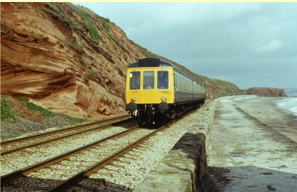
DMU along the Sea Wall near Dawlish
